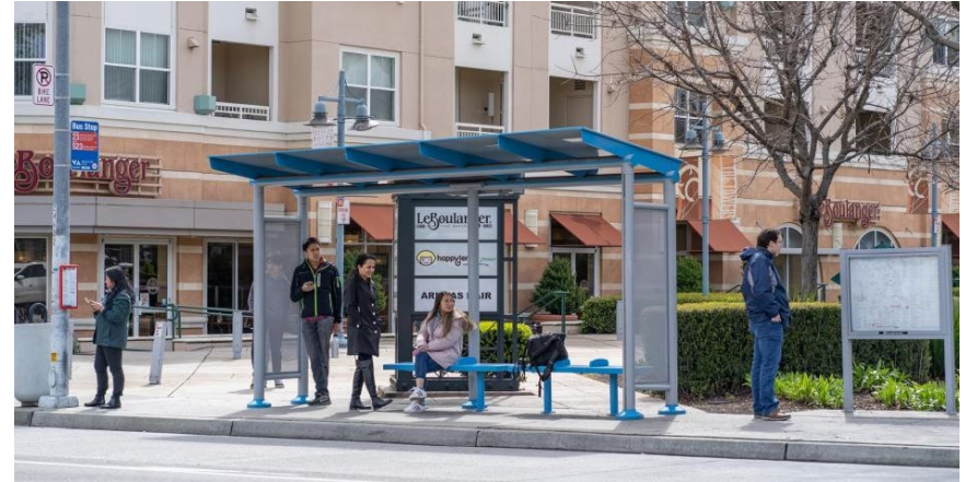
Figure 8: Rapid 523 Stop Enhancements at De Anza Boulevard
